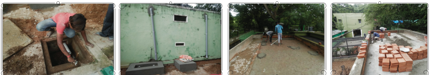
vii. Repair works at Inpatient Carnivore Wards inside Mysuru Zoo hospital
