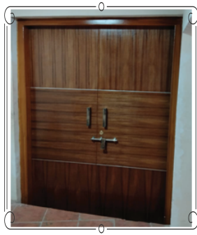
iii. Fixing of Doors to Amphitheatre Green room
