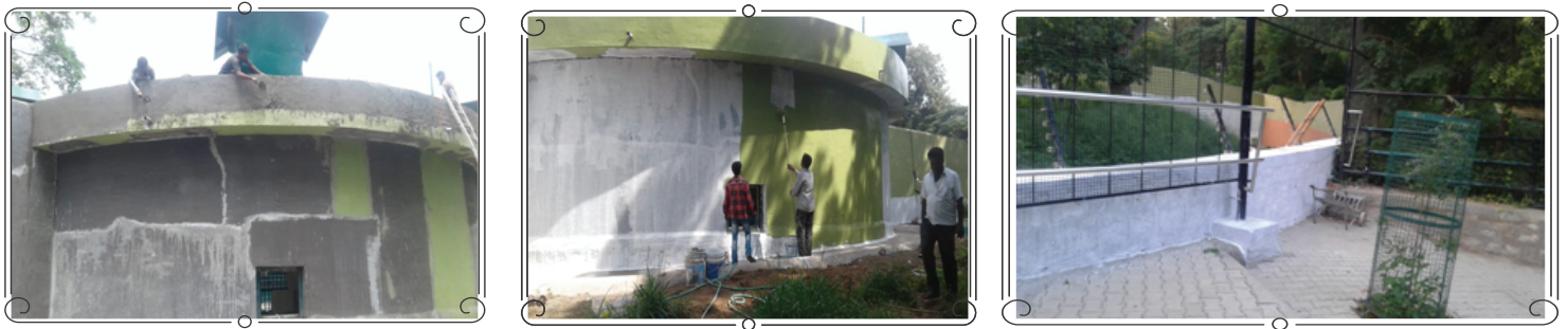
v. Painting to Fence wall & Holding Room of Hoolock gibbon
