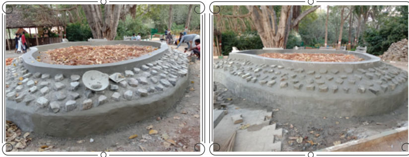
iv. Construction of Sculpture Platform near Gaur enclosure
