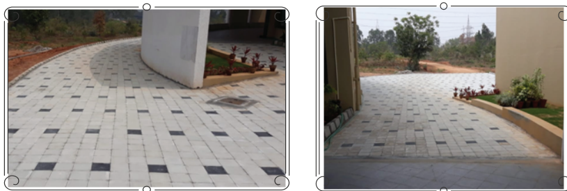
vi. Laying Interlock Pavers to Hospital building at Kurghalli
